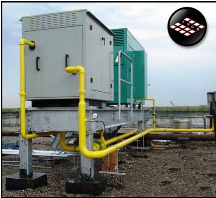
ENGBP gasPOD™ in grey outdoor transclosure feeding emergency backup generator (green transclosure).
